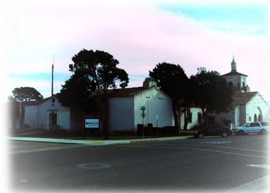
Guadalupe City Hall and Police Department
