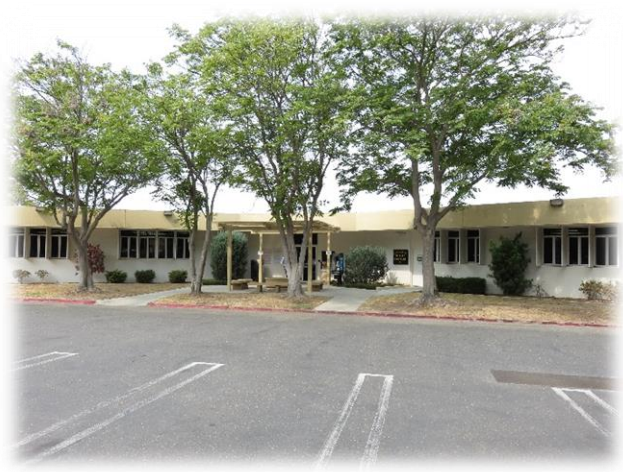
Santa Maria Substation
