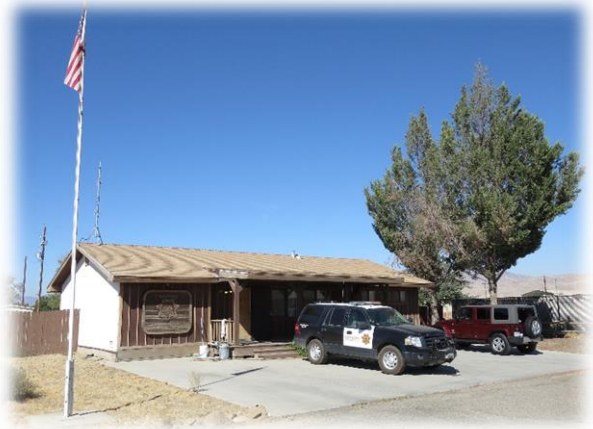
New Cuyama Substation
