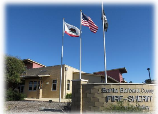
Lompoc Valley Substation
