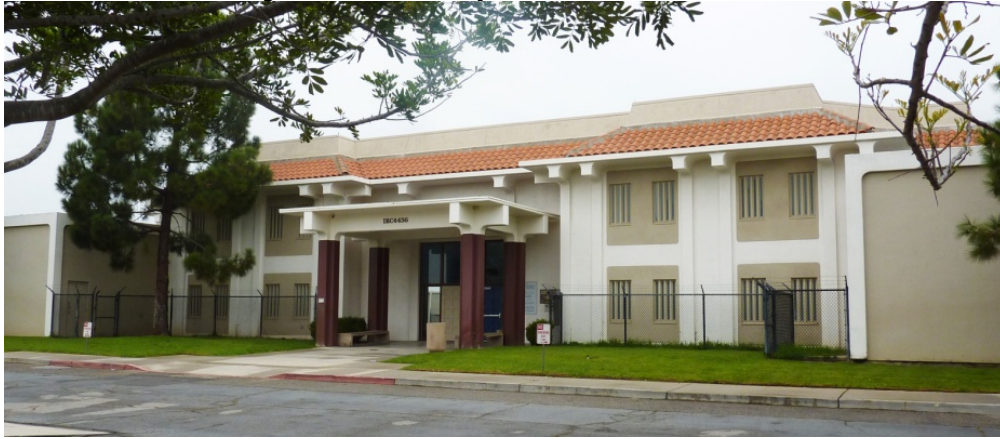
Santa Barbara Main Jail
