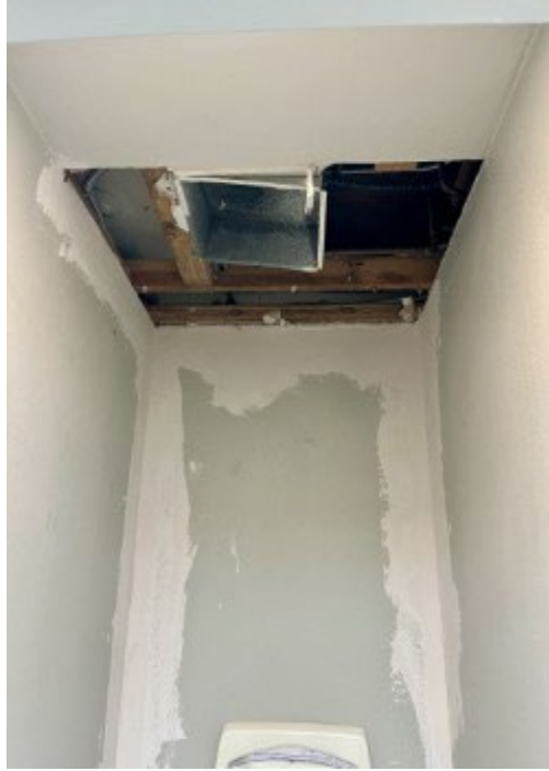
Another view of the bathroom in Bldg. 1
