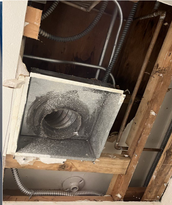
View of the bathroom ceiling in Bldg. 1
